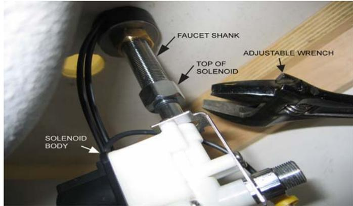
Connect the two faucet wires with the solenoid wires. The connectors are color coded. If you have an AC/DC unit, there is an additional wire with black connector coming from the top of power module that needs to be connected to the transformer provided. (not shown)
