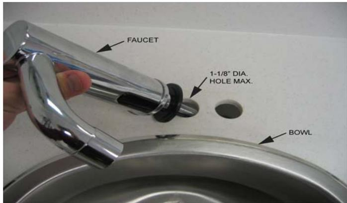
If you have a Deck Plate (either 4" or 8"), first position the gasket and the Plate on the counter top and then insert the faucet shank through the hole.
