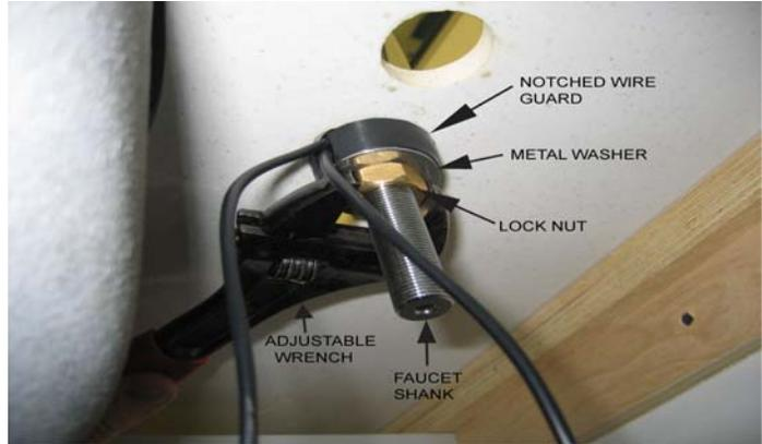
Install the solenoid by engaging the thread by hand first and continuing to tighten with an adjustable wrench (you will need to hold Faucet on top to prevent rotation). Do not overtighten and don't use any sealant. **DRY CONNECTION ONLY.**
