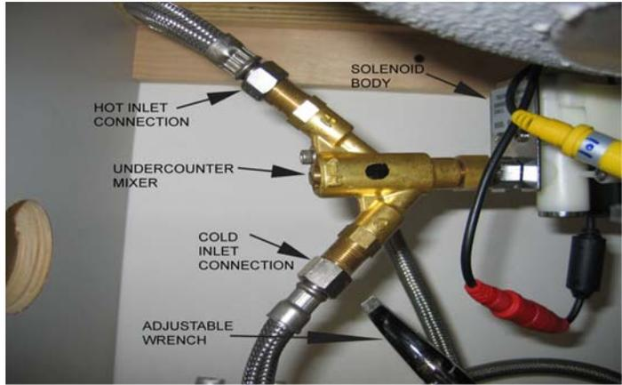
After connecting to supply lines, turn on the water and activate the faucet with your hands, checking for leaks. Adjust water temperature by rotating the screw on the UCM to your required temperature.
